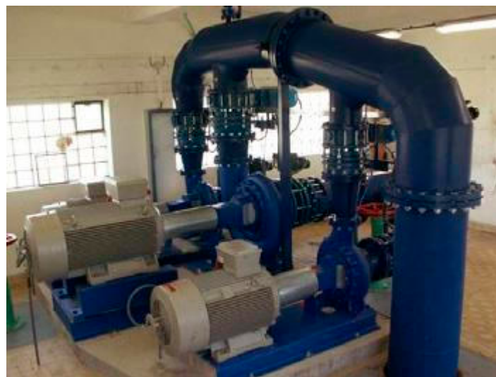
Figure 5. SHPP on a duct feeding untreated water into the water treatment plant [40].
